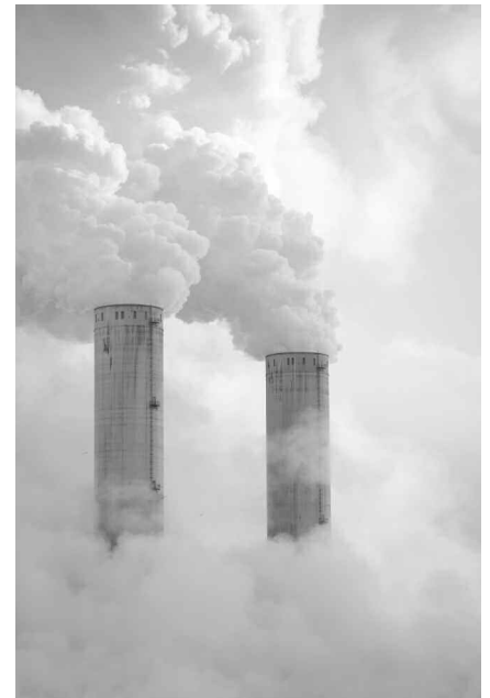
To meet local pollution standards some smoke stacks were built up to 1,000 feet high rather than installing scrubbers.
